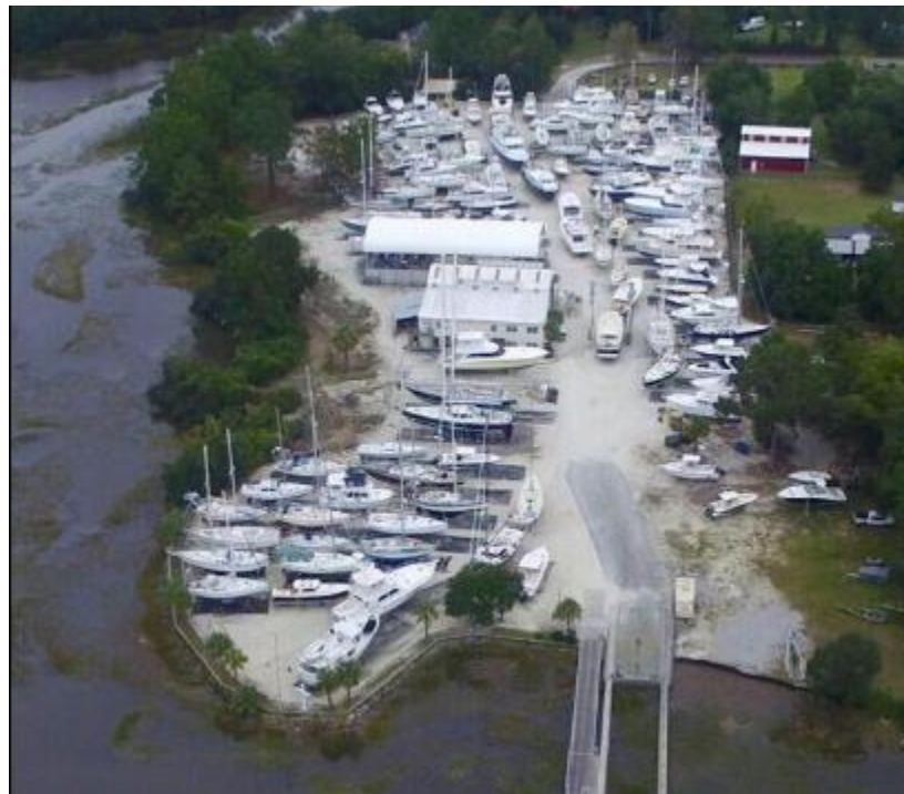
Figure 5.2: Aerial View of the Charleston City Boatyard during Hurricane Matthew (Charleston City Boatyard Interviewee, 2018)
